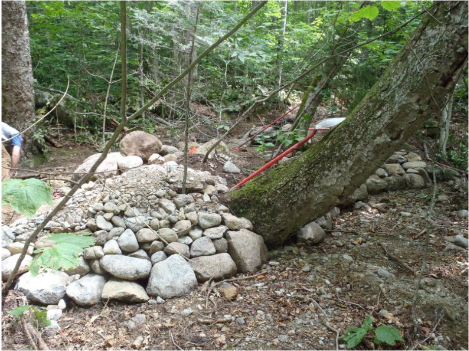
Stones used to stabilize a bank affected by an uprooted tree.
