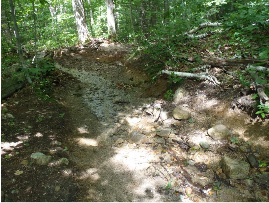
Erosion created by Tropical Storm Irene
