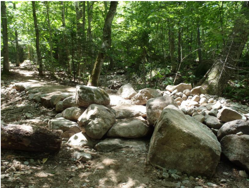
Three stone stairs built at the entrance to the reroute on the Old Bridle Path.
