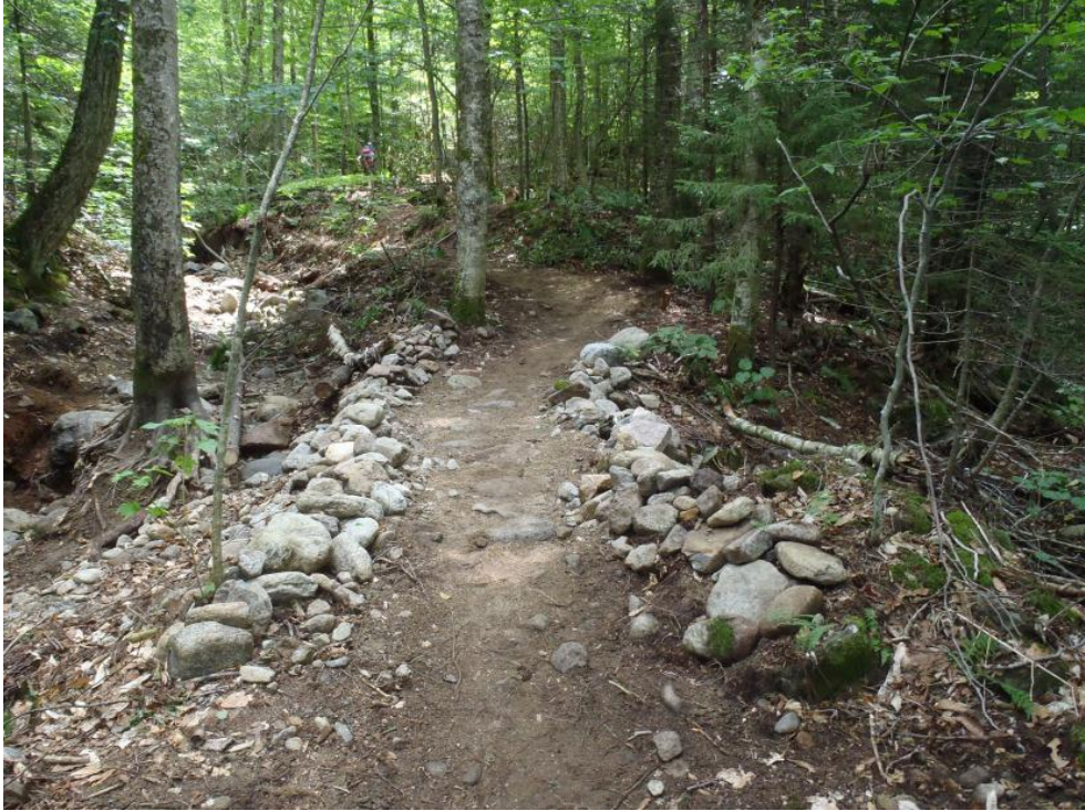
Approximately 30 feet of "turnpiking" on the Old Bridle Path reroute.
