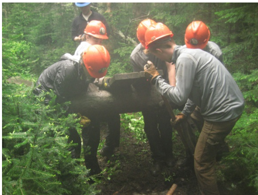
4-Week Leadership & Conservation Crew Installing Bog Bridges
